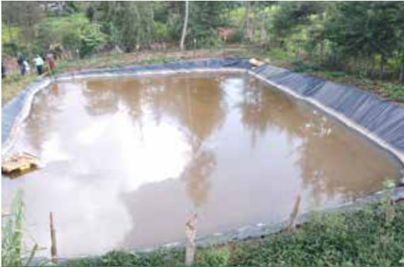
Damlining a water conservation and harvesting technique being implemented by Farmer Service Centre (FSC) Beatrice Kinyanjui in Nyandarua County.
